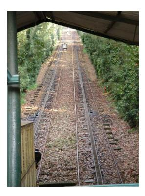
This funicular, which had a great impact at its time, is the oldest in the world powered by water ballast and still in regular service: water is loaded into the car at the top of the hill, which weights it down as it slides to the bottom, at the same time drawing the lighter, drained car up the hill, where the process starts all over again. The drained water is used for irrigation.
